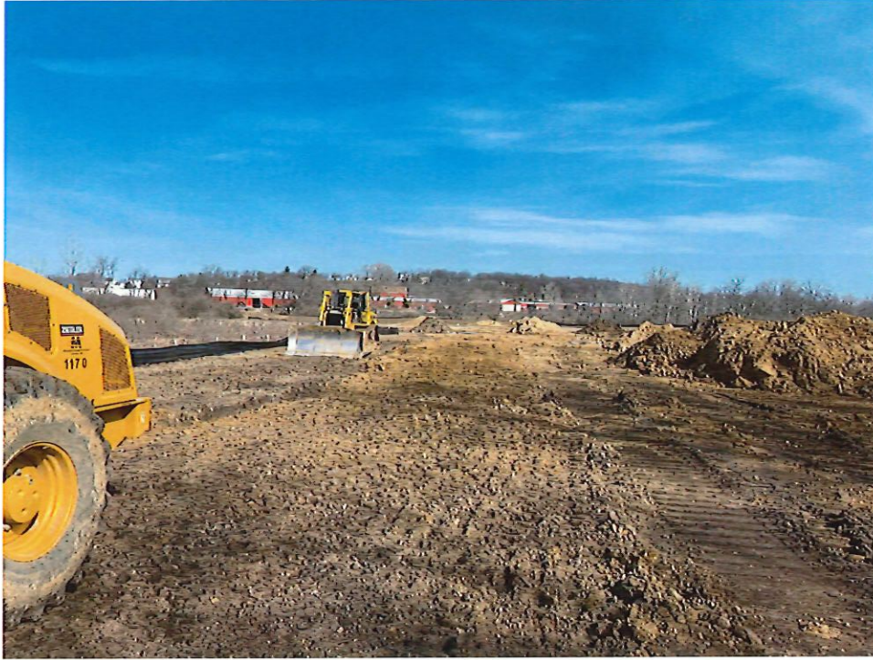
West of Goose Lake Facing North
