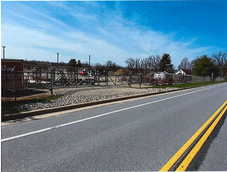
Existing Gate and base Course
