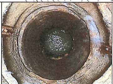
SITE PHOTO B - MMMSD MH12-106 INTERIOR
