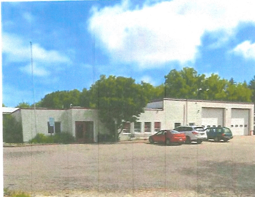
Front view of building
