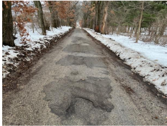
Flint Lane Facing South
