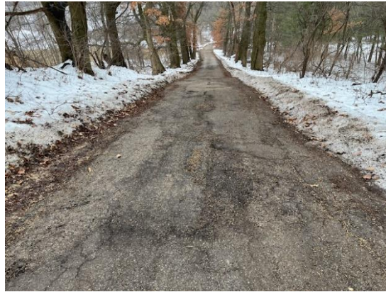
Flint Lane Facing South
