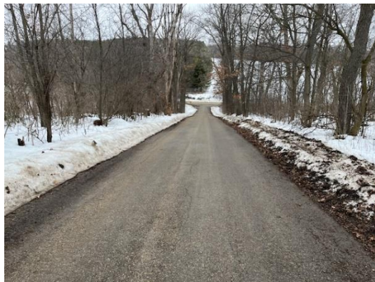
Flint Lane section Paved in 2020 facing North
