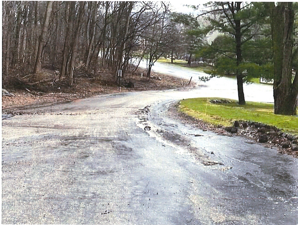
Shagbark Ct. Asphalt curb and drainage gutter 4-3-23
