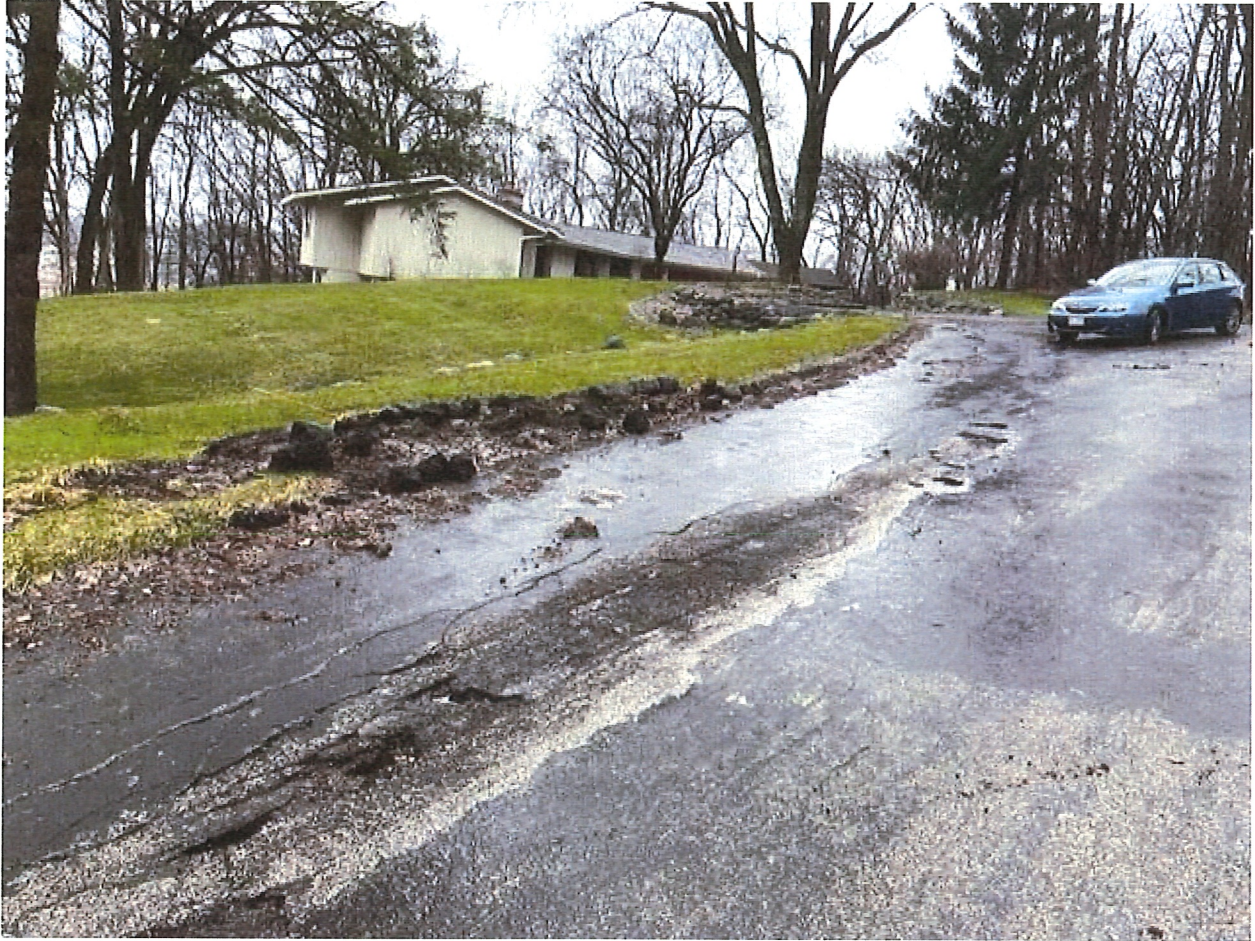
Shagbark Ct. Drainage gutter and asphalt Curb 4-3-23
