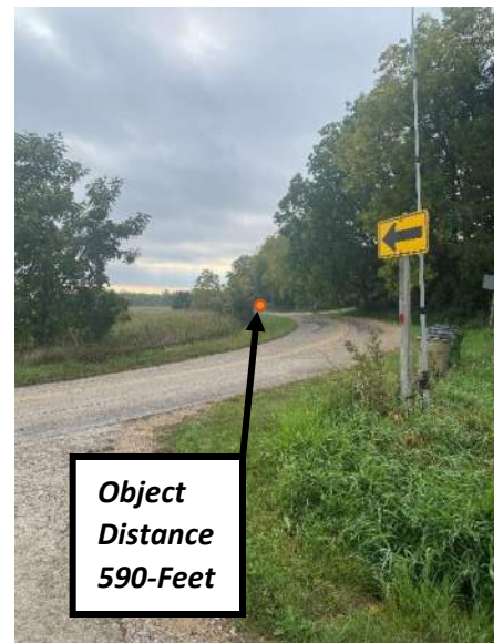
Appendix C- 12) 35 mph posted speed, desirable passenger car ISD from the South. 590-Feet
