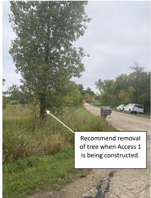
Figure 6: Uninterrupted Sightlines to the North, Beyond 785-Feet.
