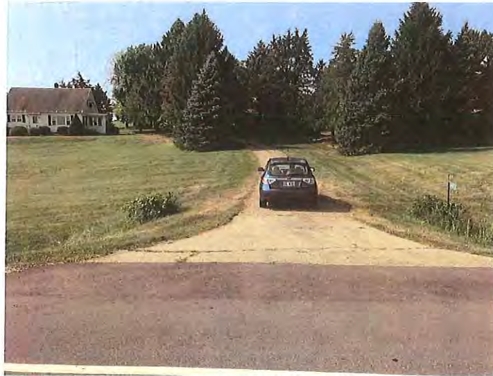
Existing Driveway on CTH M to be removed
